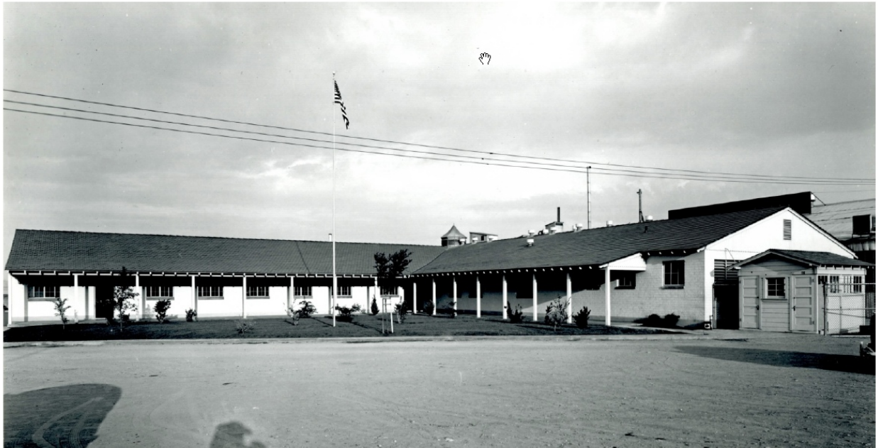
BUILDING 100 IN THE DATE STREET COMPLEX – ORIGINAL:
